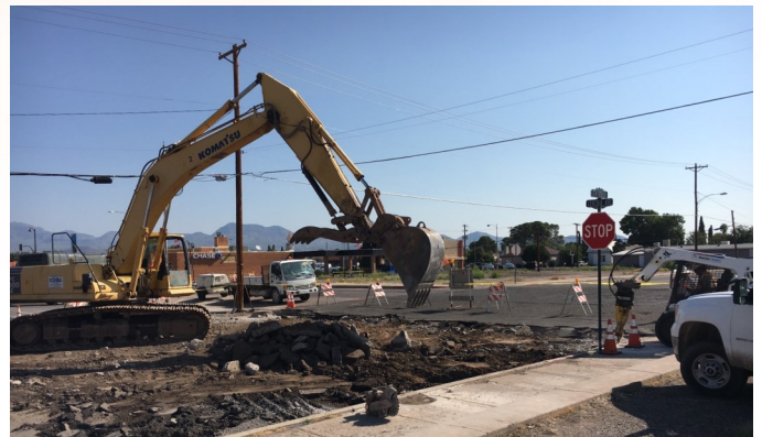
Photo of beginning construction of Central Avenue Project
